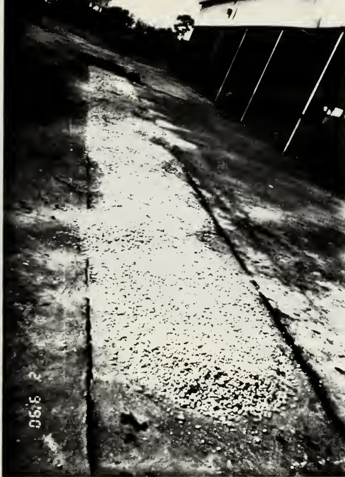
Figure 2.3 Partial Coarse Aggregate Placement
